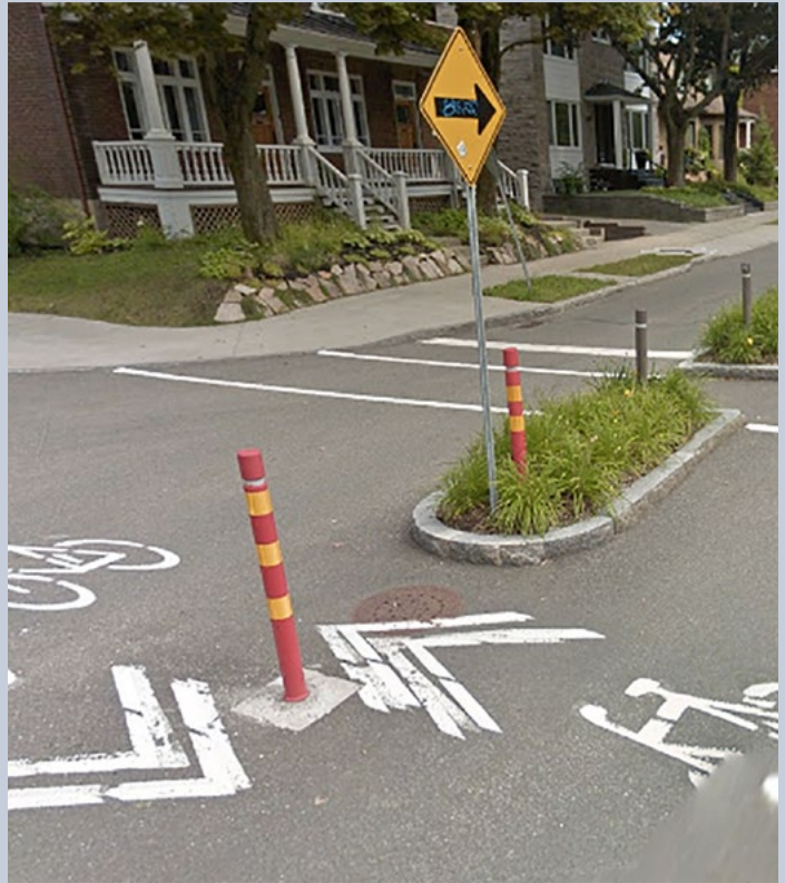
Figure 24: Bike-through median: Père Marquette Street, Québec City, QC (Photo: Google Maps)
