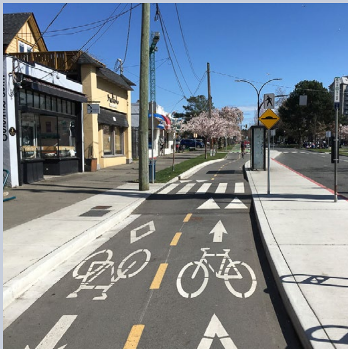
Figure 22: Concrete curb/median protected cycle track: Pandora Ave, Victoria BC (Photo: Dylan Passmore)
